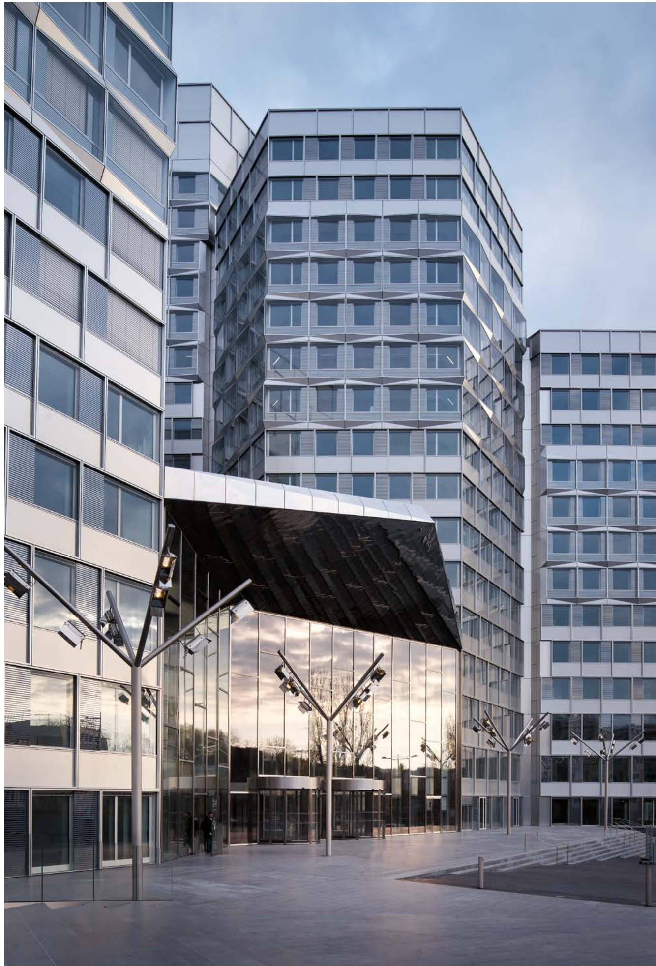
58 CityLights Büros, Paris (FR), Dominique Perrault Architecture
